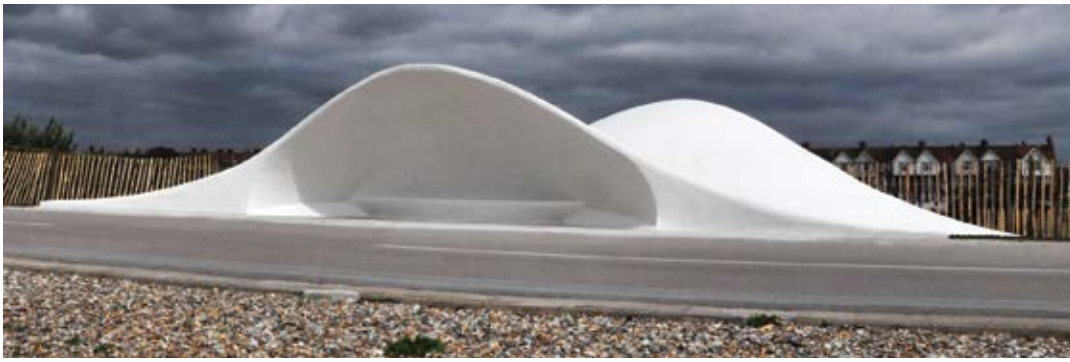
Stage and shelter (Photo courtesy Flanagan Lawrence)
