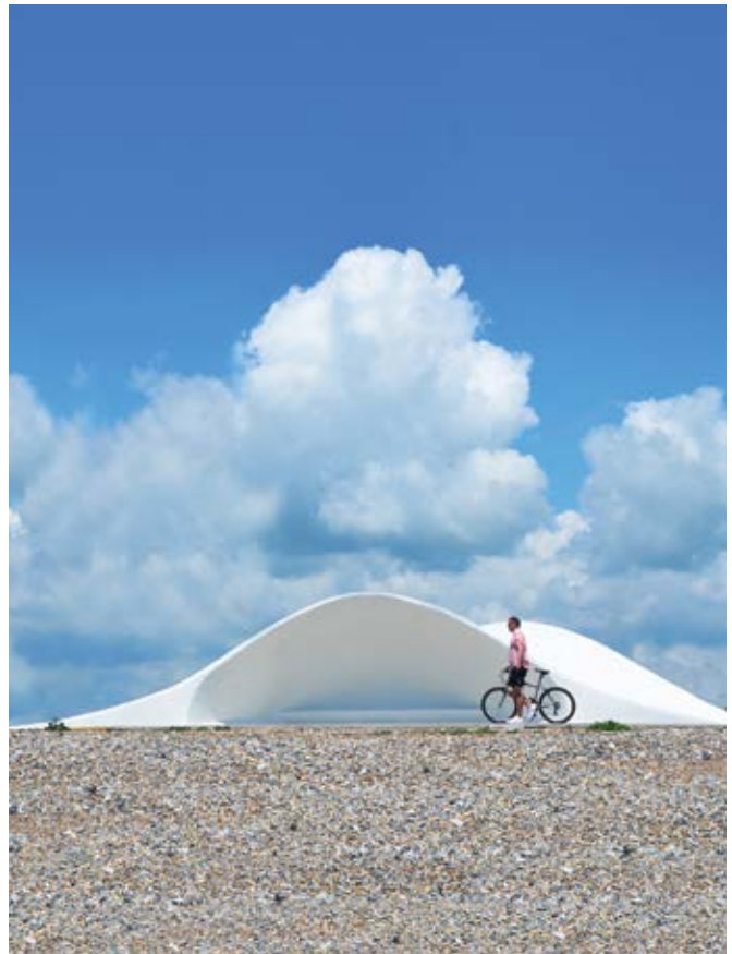
Shelter (Photo courtesy Flanagan Lawrence)
