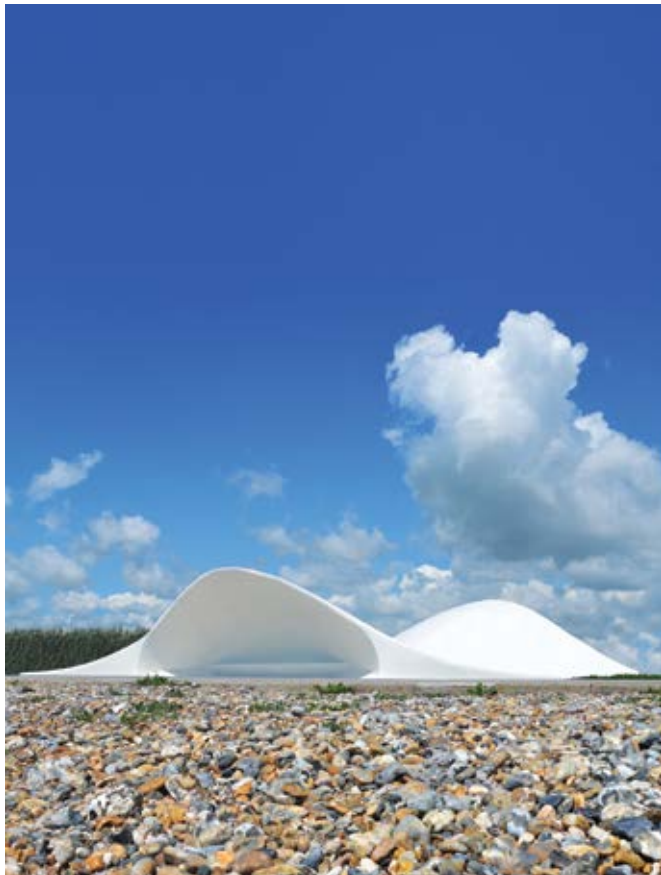
Stage and shelter (Photo courtesy Flanagan Lawrence)
